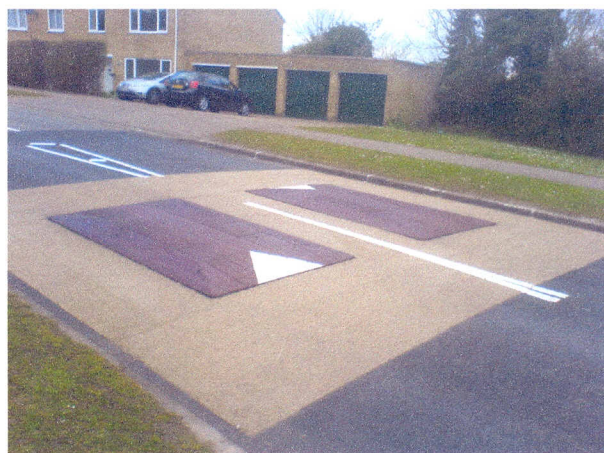
An illustration of the type of cushion to be used in Ickleford; these are 65mm high. Exact locations and width of cushions will be confirmed during the design process. This example was installed in January 2008 in Knightsfield, Welwyn Garden City
